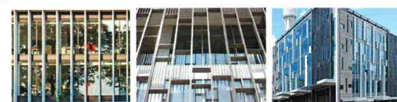
3. PRECAST CONCRETE BLADE & ALUMINUM SUNSHADE
