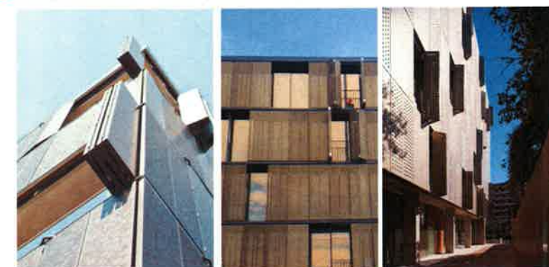
2. BI-FOLD PERFORATED METAL SCREEN
